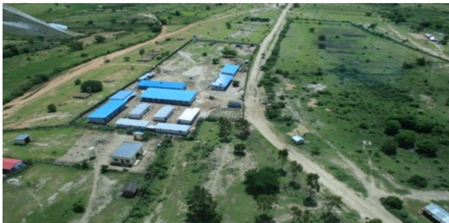
Fig 2. The new Clinic in Fotadrevo, Madagascar. A second phase is planned on this land after the functionality of the present clinic is appropriately documented and financing can be assured. Water supplies and waste water treatment will also be expanded.
