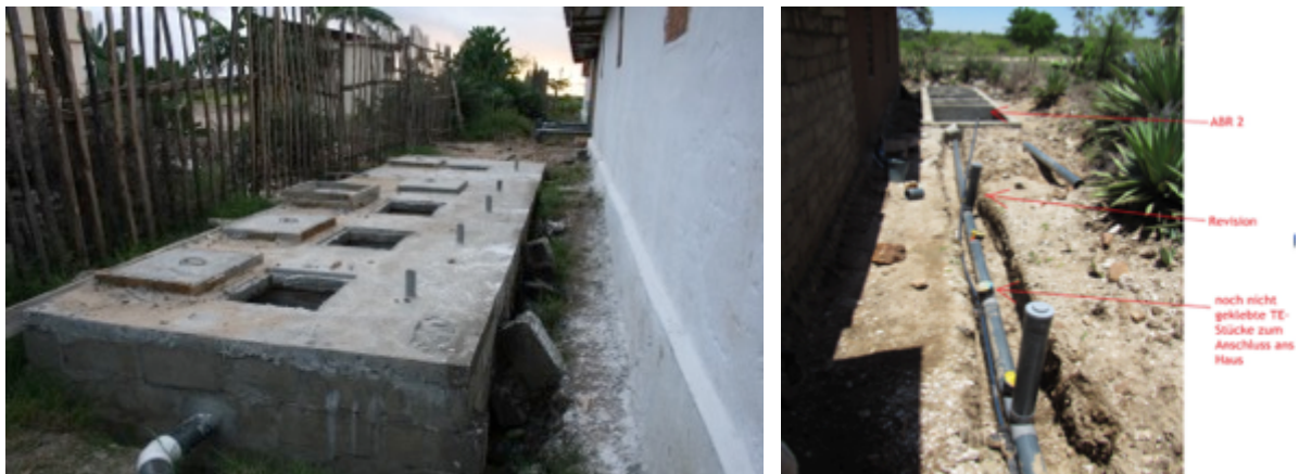
Figure 7/8. Five Chamber Abiotic Batch Reactor Unit (ABR) used for the collection and partial treatment of the waste water.
