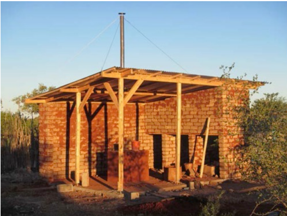
Figure 17. Incineration unit after completion Benefits
