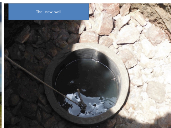
Figure 4. View of the new well.
