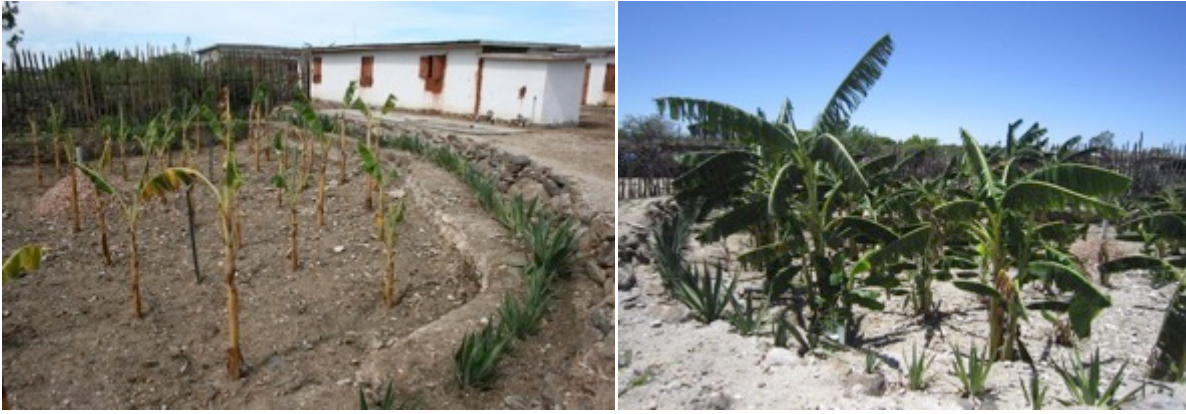
Figures 11/12. The evapotranspiration bed with banana plants at end of construction and 6 months later
