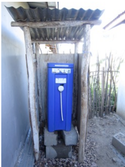
Figure 5. Public access – membrane-filter-PAUL used for the hygienisation of drinking water
